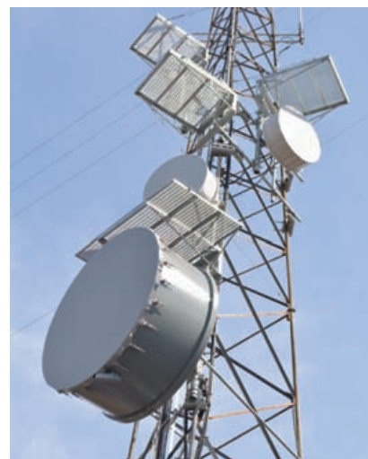
The microwave dishes at Central Hudson's headquarters communicate with remote dishes like these, on commercial communications towers. These towers facilitate communications and relay data from Central Hudson's fixed assets.
