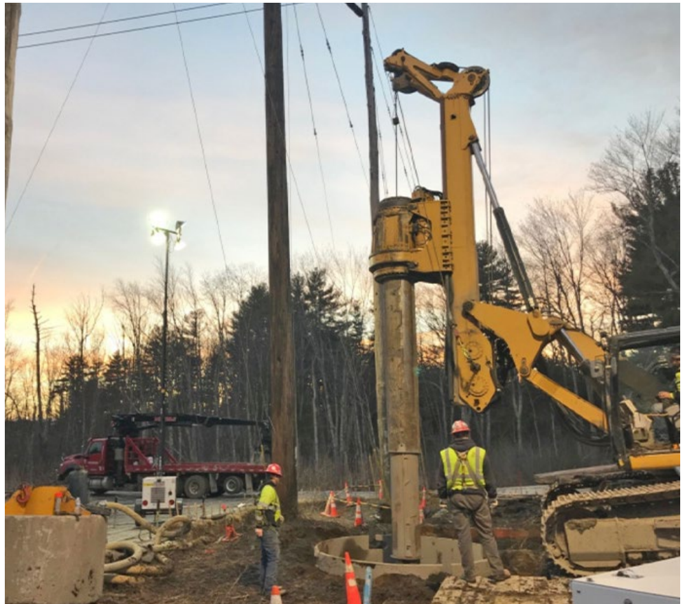
Construction of 345-kV transmission line foundations | Michels Power
